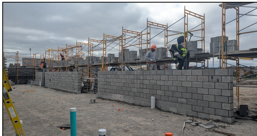
Load bearing masonry walls being erected.
